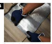
Pressing firmly with both hands, bend the flashing to form to the contour of the roof tiles.
