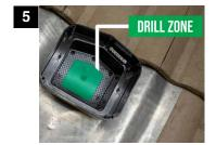
Place the JB-2 base into the opening in the flashing. Using a drill bit, drill through the box & roof simultaneously within the approved 'Drill Zone'. Verify penetration hole(s) are on either side of a rafter but not over or through a rafter/truss.
