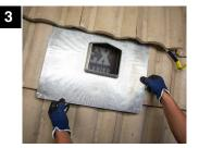
Insert aluminum flashing with the top edge underneath the row of tiles above, center pentagon flashing in opening.
