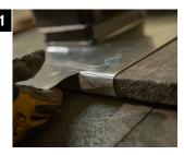
Use a pair of tin snips to snip the bottom edge of flashing on each side (min 1" wide) creating a tab. Tuck tabs under adjacent tiles to help keep the replacement flashing flush to the roof.
