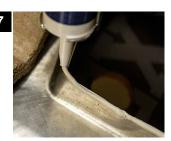
Apply a generous bead of sealant to flashing sidewalls.
