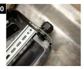
Populate the JB-2 using the appropriate wire connectors, terminal blocks, or other needed components that are suitable for the intended purpose.
