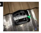
Secure the JB-2 to the roof decking using (5) #10 x 1-1/4" Phillips pan head screws (provided). Install outdoor-rated, UL 514B, NEMA 3R approved fittings and/or strain reliefs to the EAST, WEST and SOUTH side walls of JB-2 and complete wiring installation. Up to 1" raintight fittings are all acceptable. Clean off all burs.
